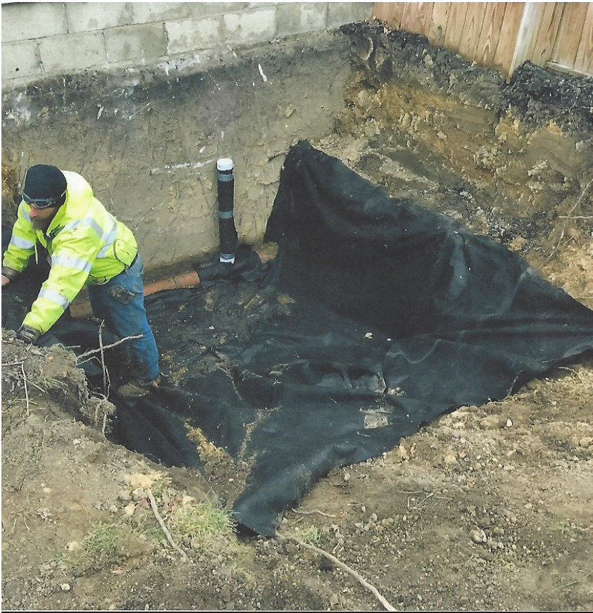
PRO member, Unified Construction, diligently helping with the Rachel K. Project
